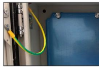
Grounding screw More aesthetically pleasing and safer
