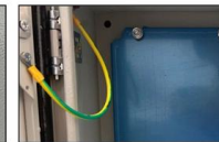
Grounding screw More aesthetically pleasing and safer
