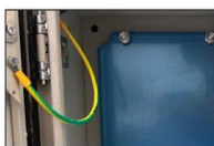
Grounding screw More aesthetically pleasing and safer
