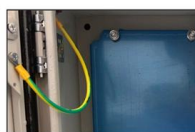
Grounding screw More aesthetically pleasing and safer
